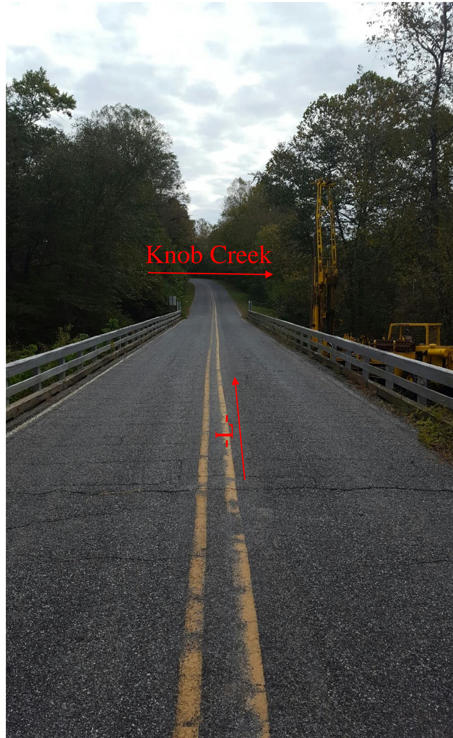
Photograph No. 1: Looking at End Bent 1 toward End Bent 2
